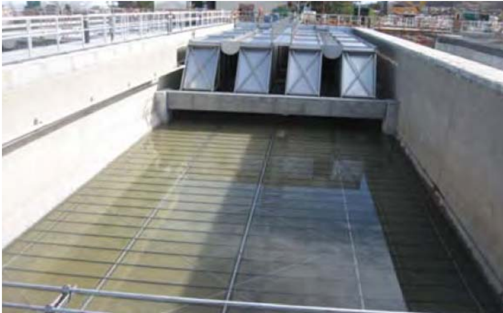
Figure 5-4 Sedimentation Basin with Plate Settlers
