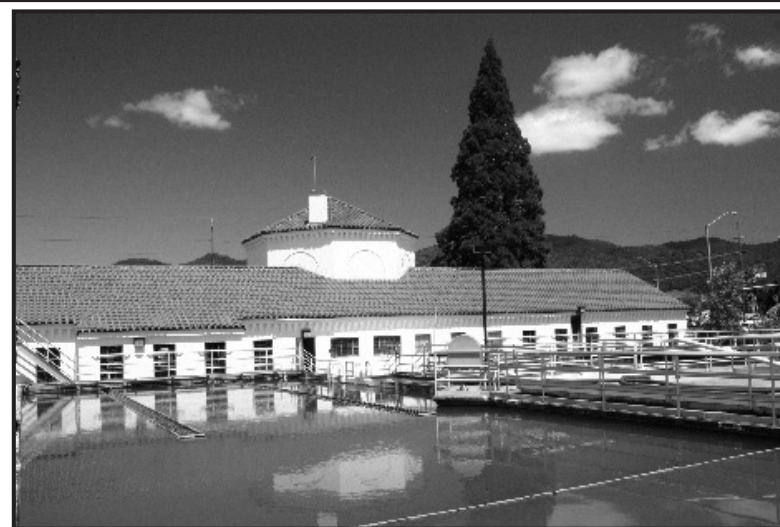
THE CITY’S AGING WATER TREATMENT PLANT WAS BUILT IN 1931.
