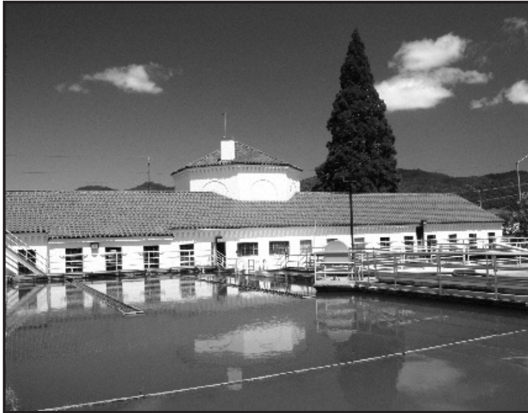
THE CITY'S WATER FILTRATION PLANT AND POND.
