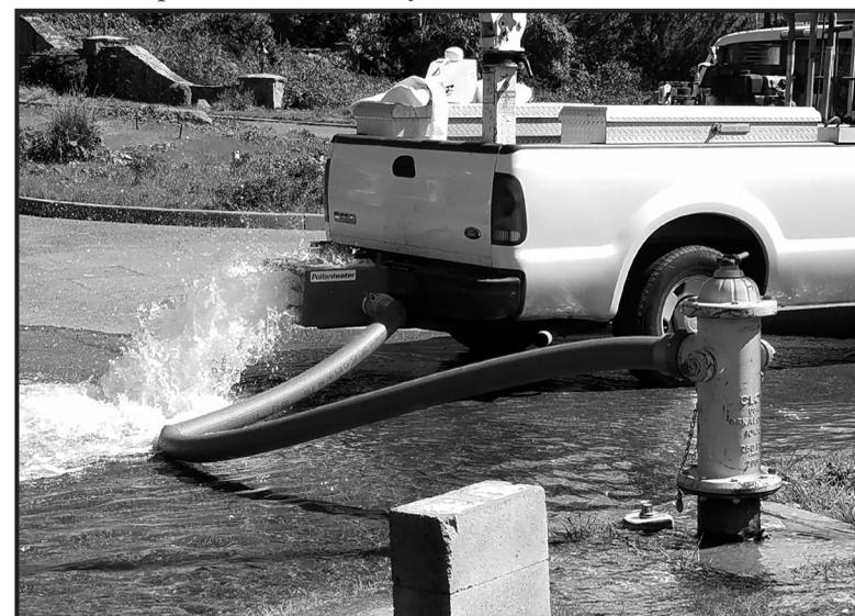
**CITY CREWS CONTINUE UNIDIRECTIONAL FLUSHING OF THE CITY'S 188 MILES OF WATER PIPING.**
